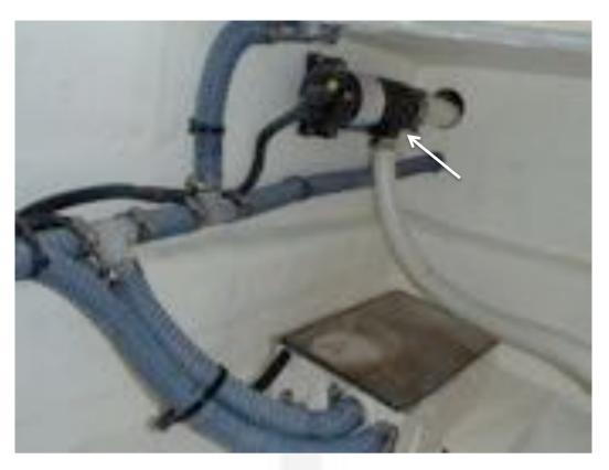
Image of the macerator pump which was found to be defective.
